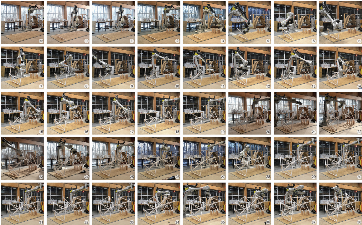
Figure 4-8: Construction timelapse collage for the Short Arch.
